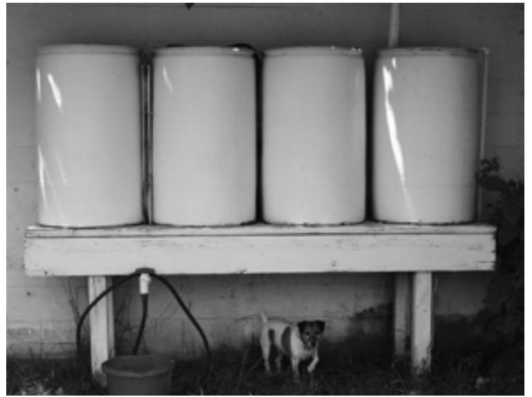
Rain Barrels: Saving rain water is a great way to save money while ensuring water for thirsty gardens in the summer. This simple four barrel collection system cost less than $100 to build. (Jack Russell is extra.)
