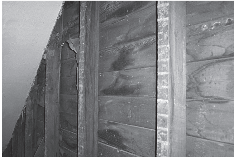
Close-up of Balloon Framing
