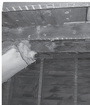
Close-up of Balloon Framing
