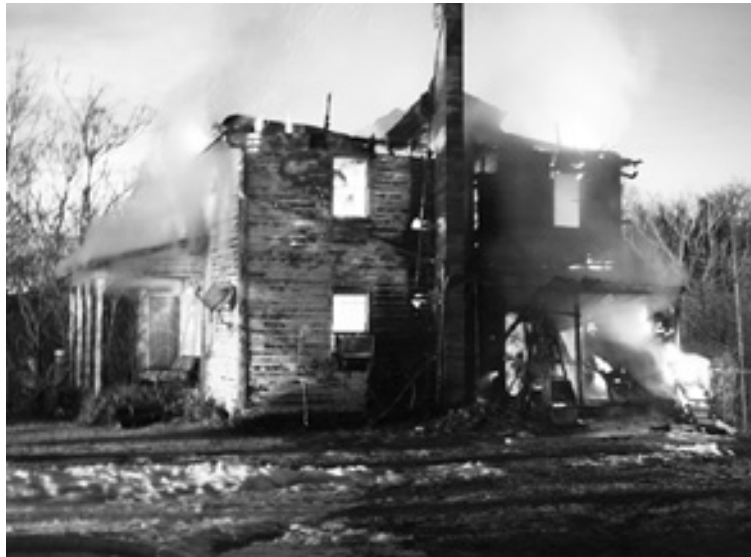
While the old Clara Harner farmhouse on Sixes Road was completely destroyed, the adjoining historic slave quarters were saved.
