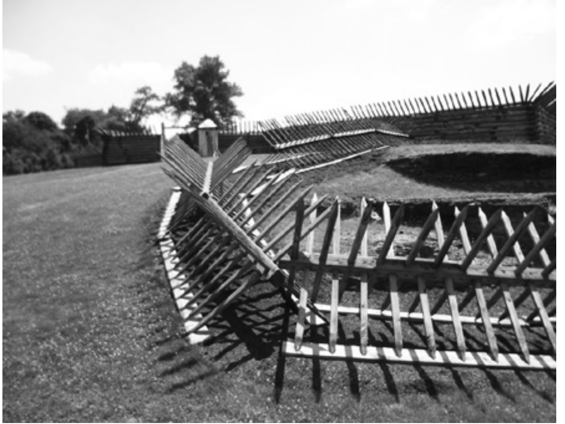
Crossed pickets in front of and on top of fort walls were effective in breaking up frontal assaults by mass troops during the French and Indian War.
