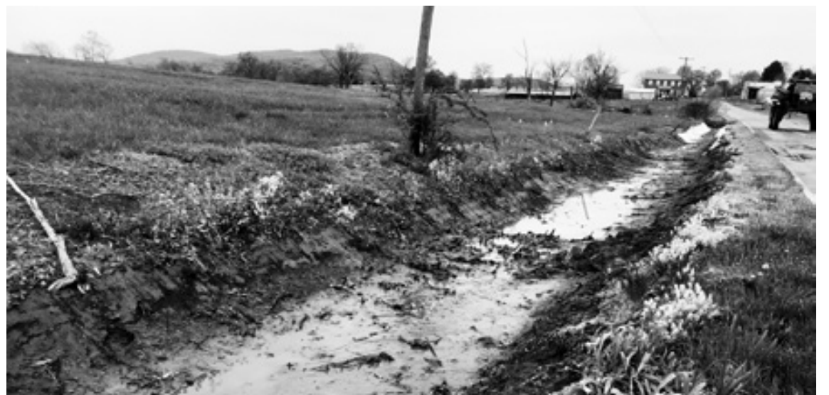
The once beautiful Riparian barrier is now a eyesore mud pit, ensuring that all runoff will now run unfiltered into Tom's Creek, increasing the pollution level in that water body. Had the destruction of this Riparian barrier been done by a farmer or a home owner, the County would more than likely have fined them and required the barrier's restoration. But because the County did the damage ...
