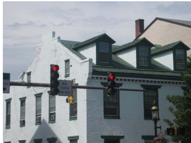
Dormers on a building at “the Square”
