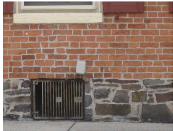
Typical stone foundation in Emmitsburg
